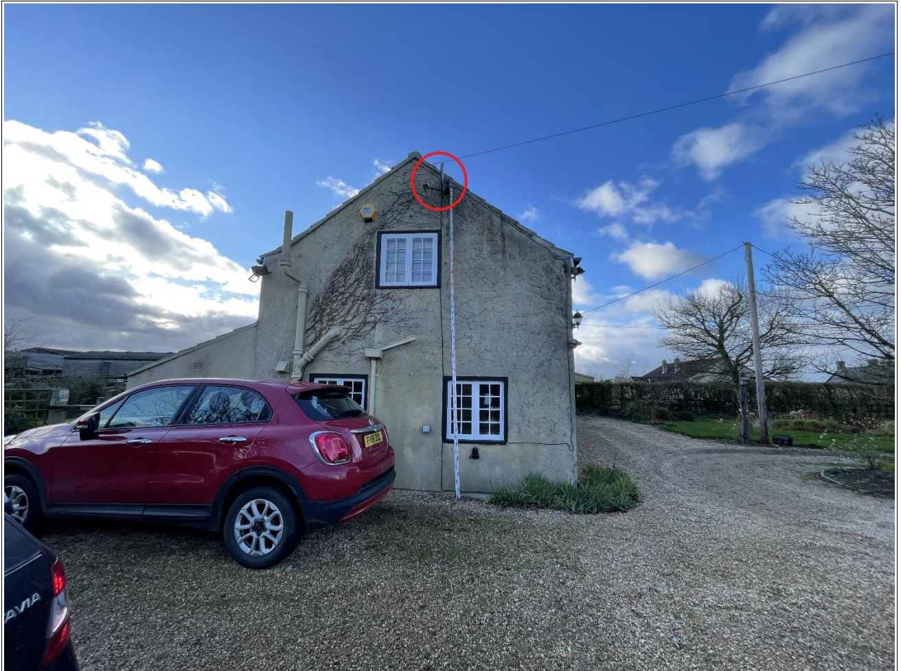
Fig. 2 Existing satellite dish
