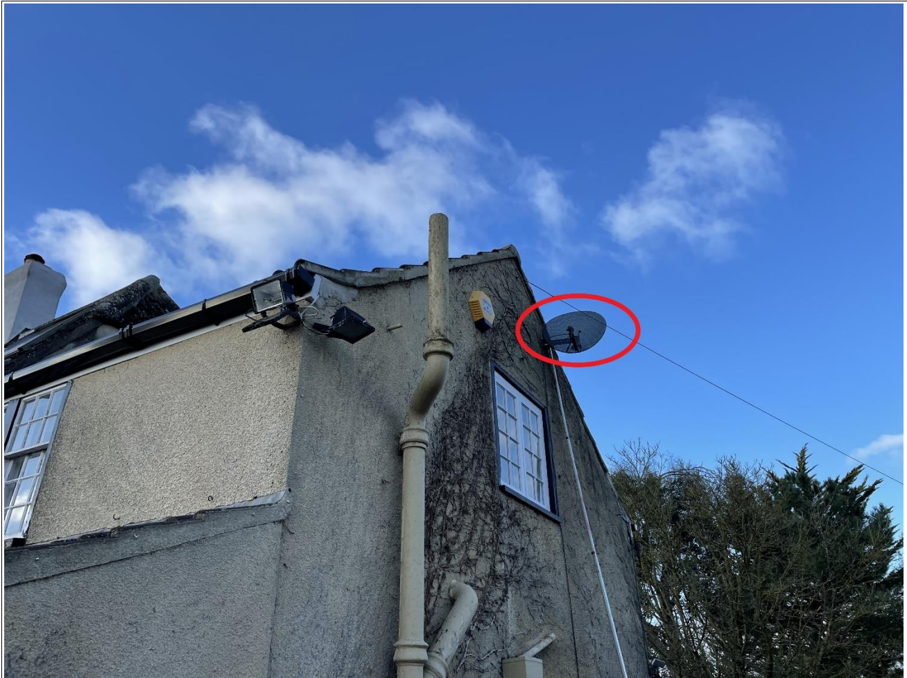
Fig. 3 Existing satellite dish
