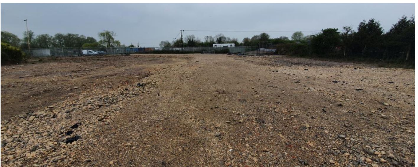
Site photos of the cleared site taken in May 2021. The demolition of the Countrywide Store was undertaken in 2020 pursuant to 19/04937/DEM
